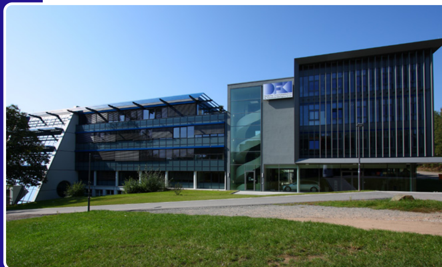
DFKI-Building Saarbrücken, Germany
